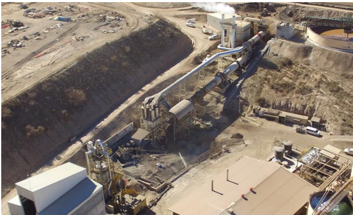
Figure 17-3: Aerial View of the Roaster Circuit
