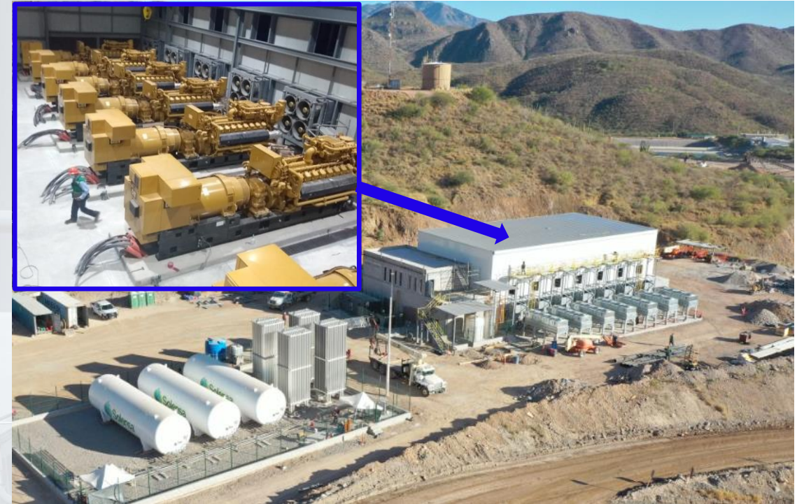
Santa Elena's new 12.4MW LNG Power Plant
