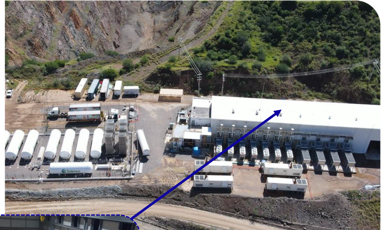
Santa Elena's 24MW LNG Power Plant
